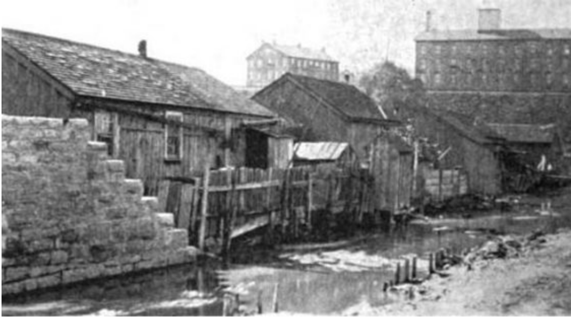
Photo 1.1: Syracuse, NY—Shanties Back to an Open Sewer. (1901)
